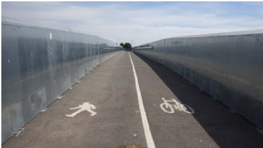
Westwood Railway Footbridge - After
